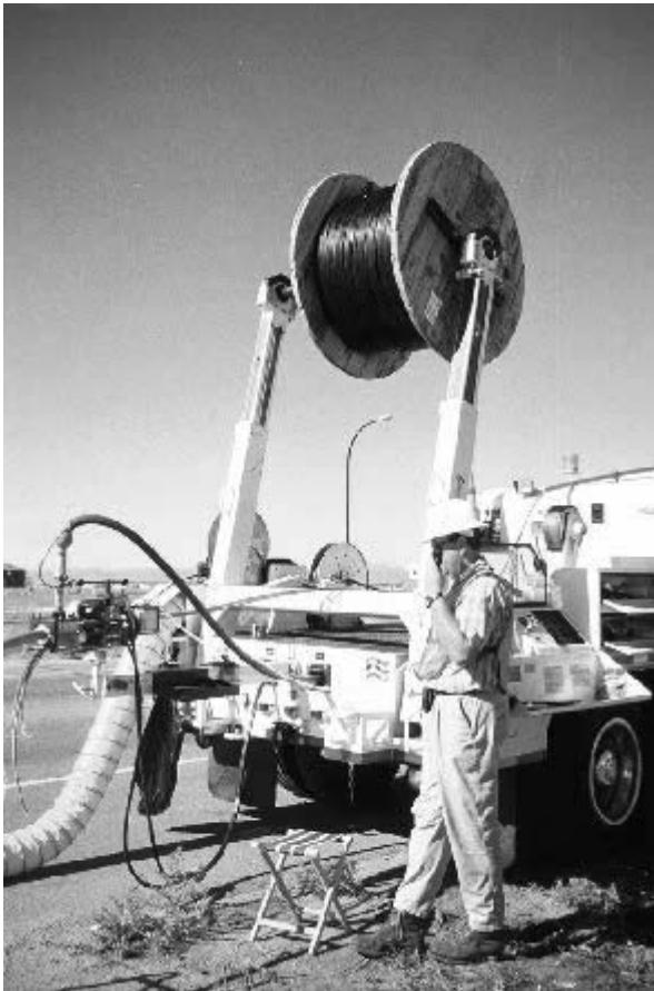
Figure 5.16. Microducts being fed into the mechanical drive of a cable jetting machine. (Photo courtesy of Sherman & Reilly, Inc.; www.sherman-reilly.com .)
